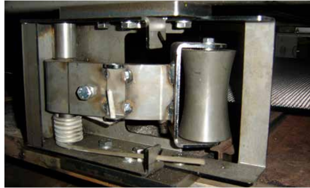
A too high tensioning of >4 bar
