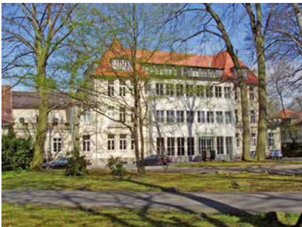
Administration building in Mülheim an der Ruhr, Germany
